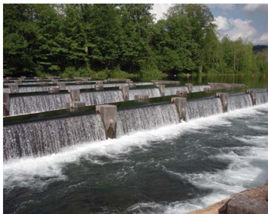
Overflowing Weir Dam
