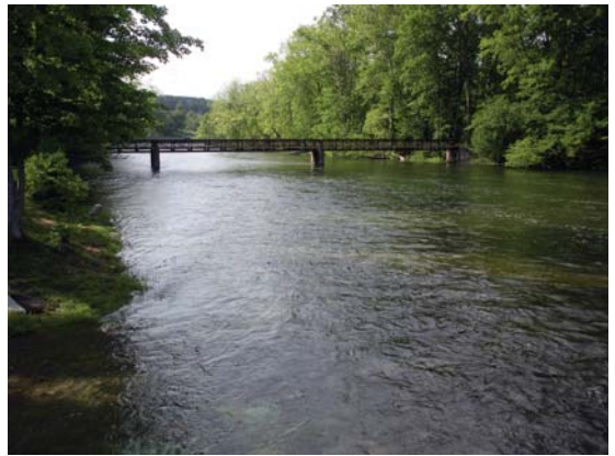
Downstream view from Weir Dam.
